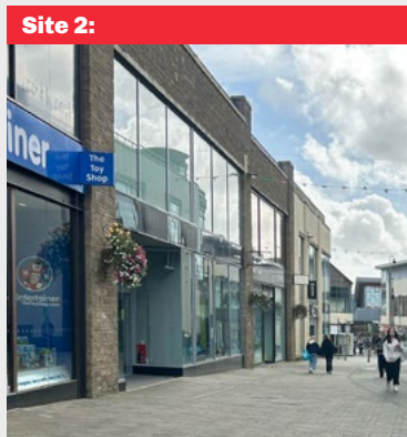
Site 2: Top End: Multiple sites available along this broad pedestrian shopping area featuring major retailers like Next and H&M. Power is available on-site.
